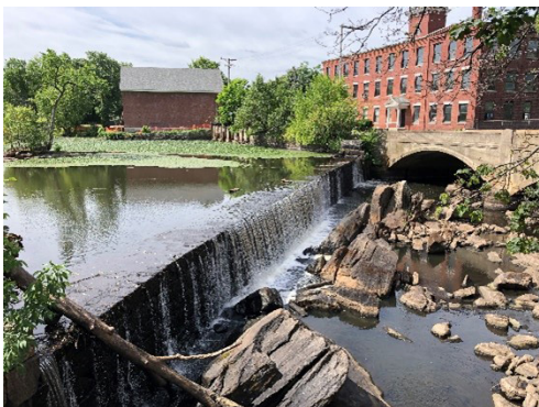
Talbot Dam is slated for removal in Billerica, MA. Credit: USFWS
