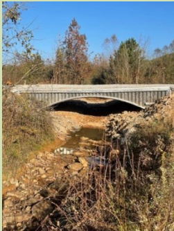
New bottomless culvert in Springville, AL. Credit: USFWS
